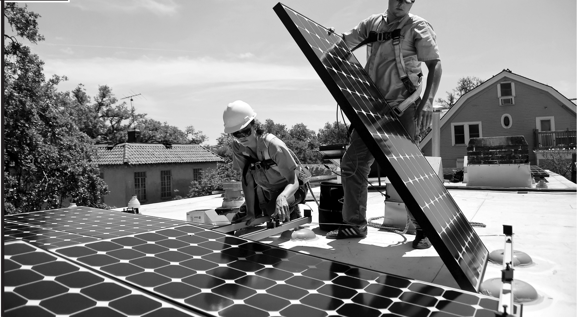
South Coast Solar technicians Lauren Craig and Micah Galy install solar electric panels at a Garden District home.
