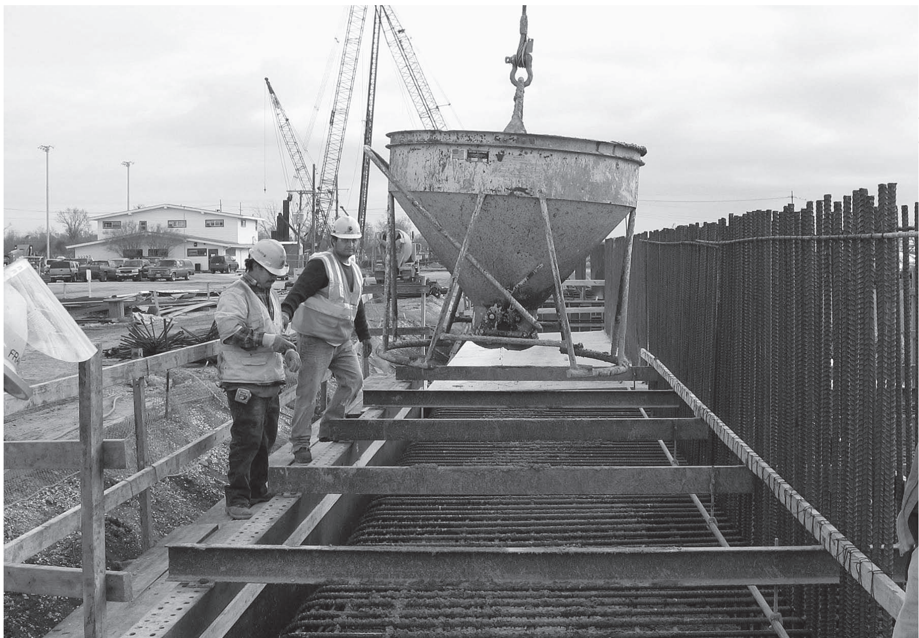
Above: Workers with Cajun Constructors monitor concrete being poured for the $250-million floodwall on the West Bank. Below: Cajun Constructors is working on the second phase of the West bank floodwall, an 8,300-foot barrier stretching from the Harvey Canal sector gate at Lapalco Boulevard to the S-curve of Old Peters Road.
