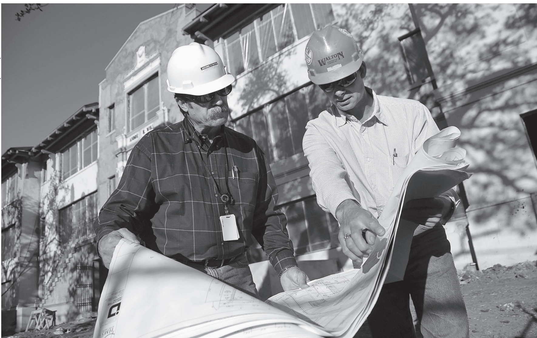
Jacobs Engineer project manager John Taylor, left, reviews plans with Walton Construction superintendent Rocky Pfeifer for the Recovery School District's Andrew Wilson Elementary School.
