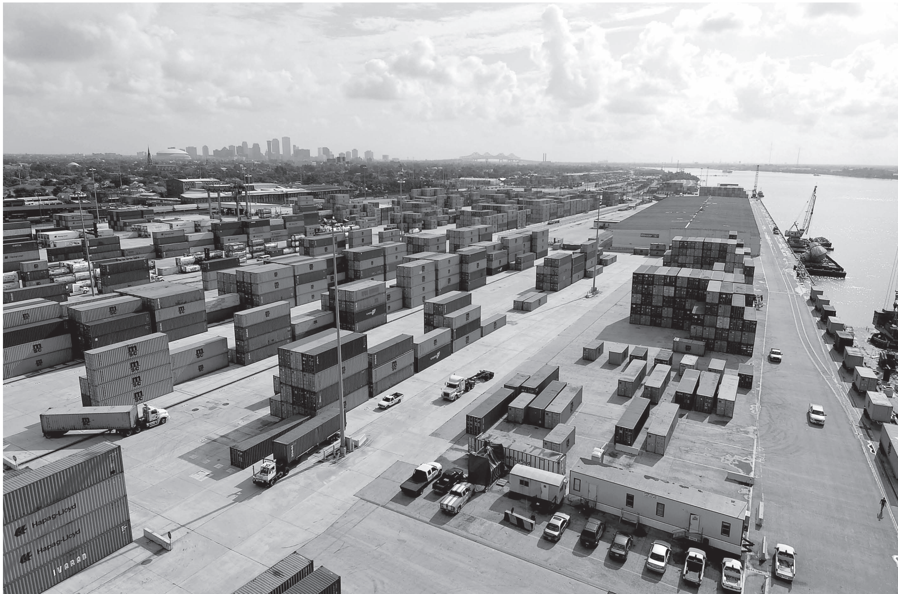
The next phase of the Napoleon Avenue container terminal includes three new gantry cranes, two of which are expected in July, additional container handling facilities and an intermodal rail yard.
