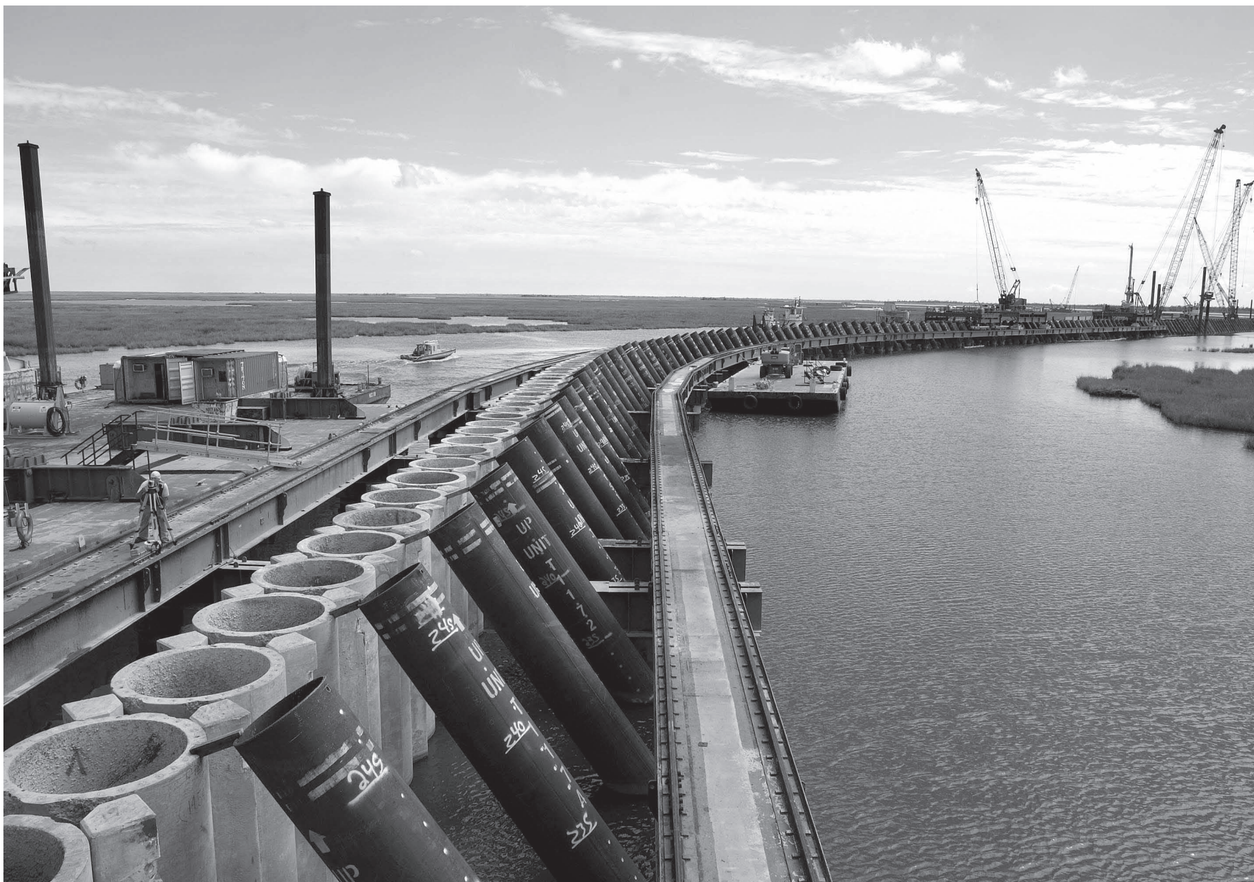
Work continues on a two-mile-long, 26-foot-high storm surge barrier near the point where the Gulf Intracoastal Waterway meets the closed Mississippi River Gulf Outlet.
