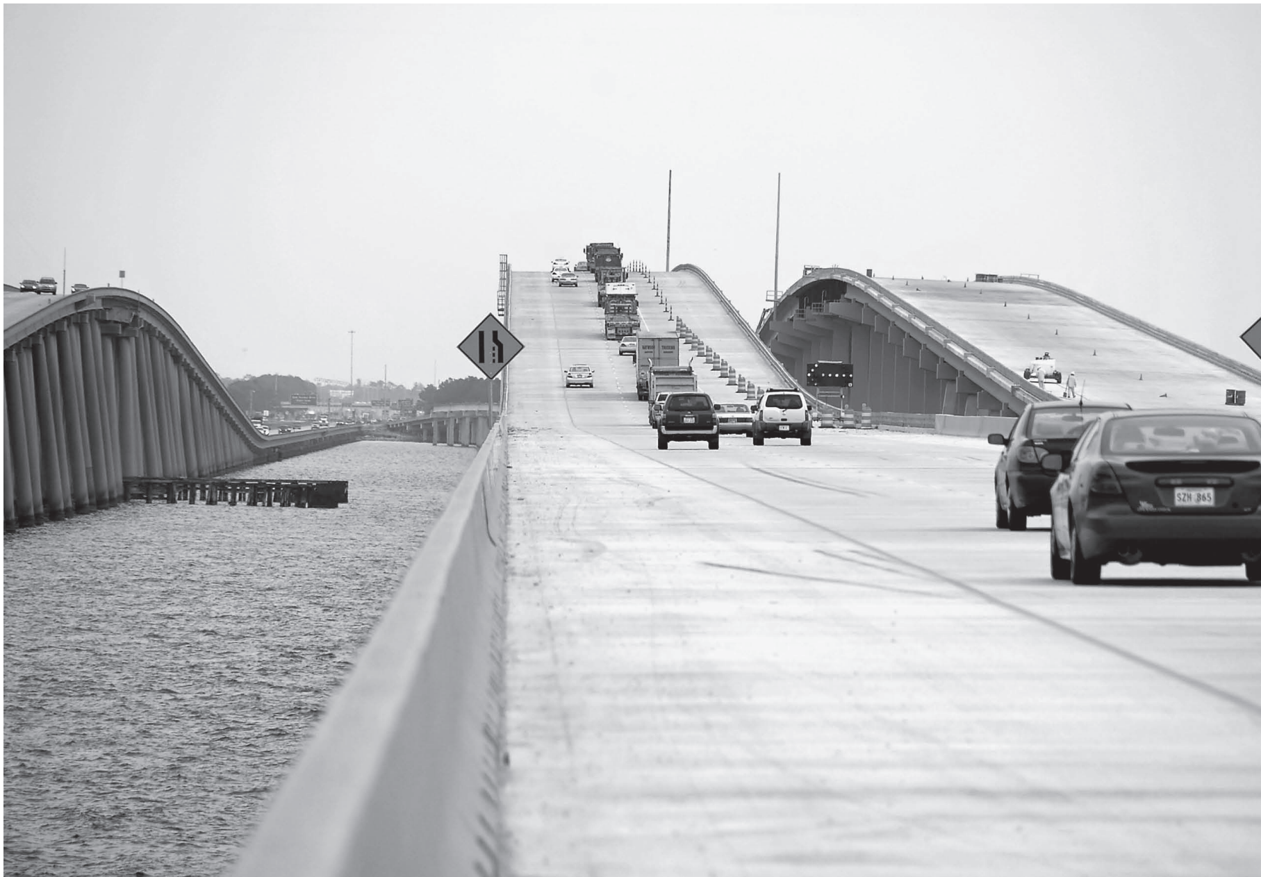
The eastbound span of the Interstate 10 Twin Span is scheduled for completion in mid-2011.
