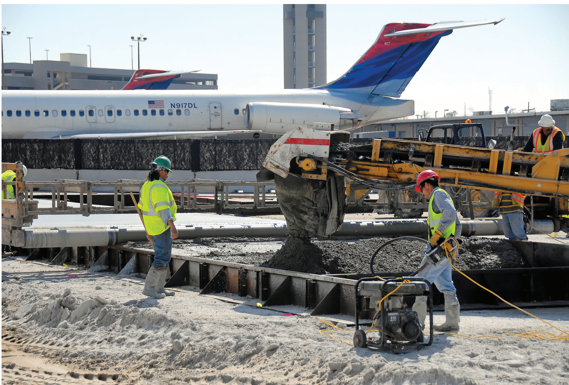
Workers pour concrete for an upgraded air carrier apron surrounding the terminal and concourses at Louis Armstrong New Orleans International Airport.
