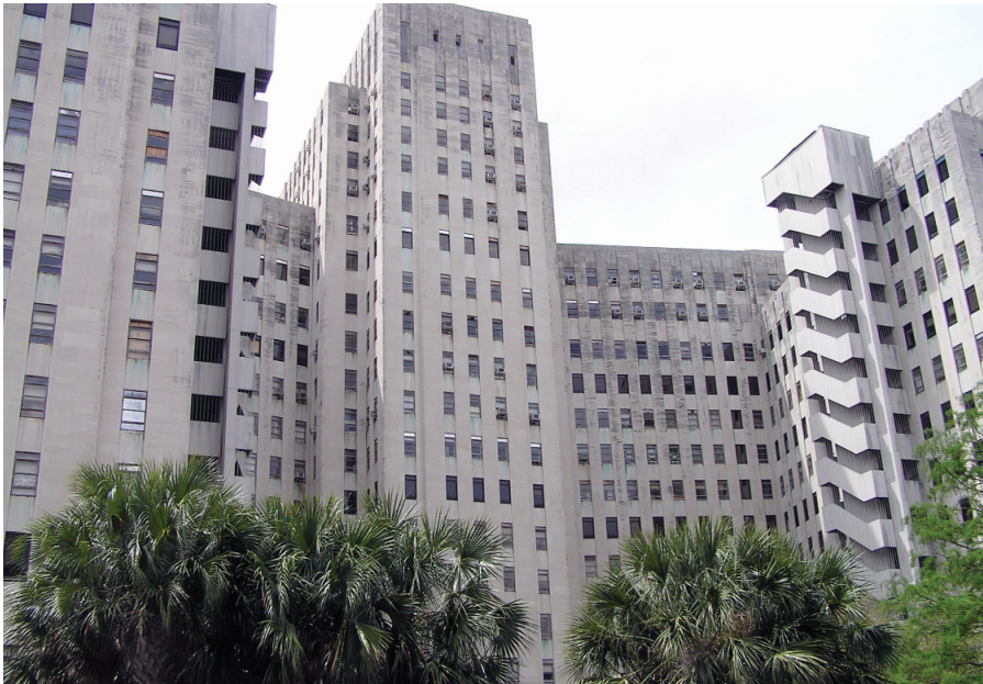
A federal arbitration panel recently ordered the Federal Emergency Management Agency to provide $474.8 million to repair Charity Hospital after the agency originally offered a repair estimate of $126 million.
