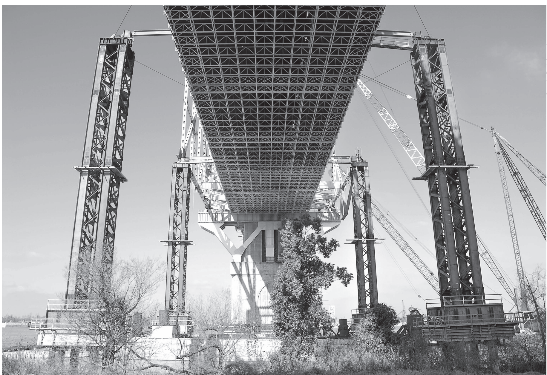
In June, workers will lift two steel trusses as part of the main span support for the Huey P. Long Bridge expansion project.
