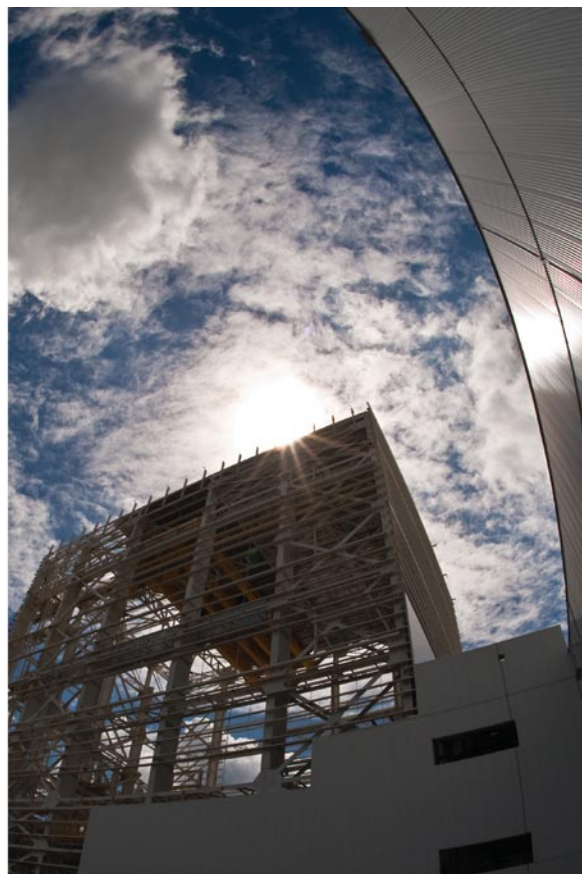
NASA VERTICAL ASSEMBLY BUILDING Michoud Assembly Facility, New Orleans, LA
