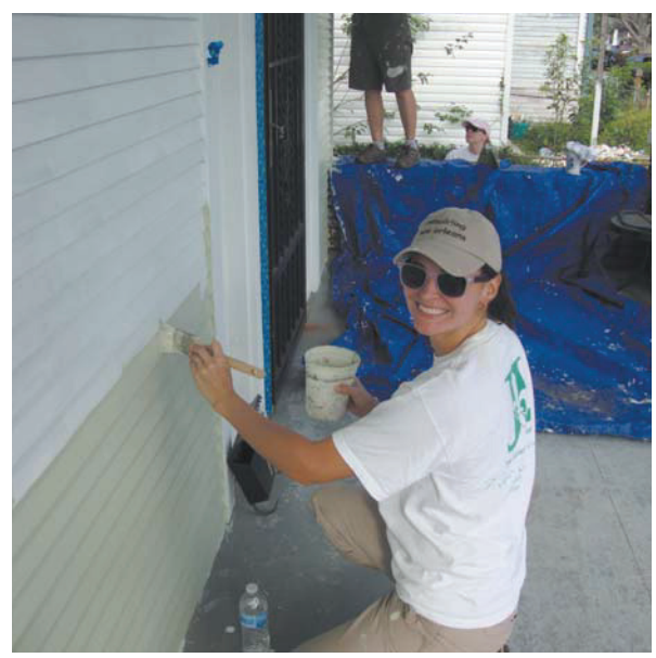
Rebuilding New Orleans
